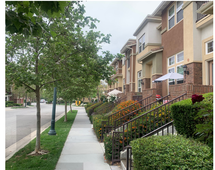
Building Setbacks. Building on right is setback approximately 10-15' from property line.
